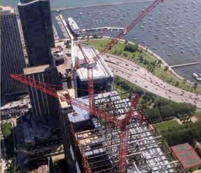
Two Potain MR 605B luffing tower cranes at the Blue Cross Blue Shield Tower vertical expansion, Chicago, Illinois.
