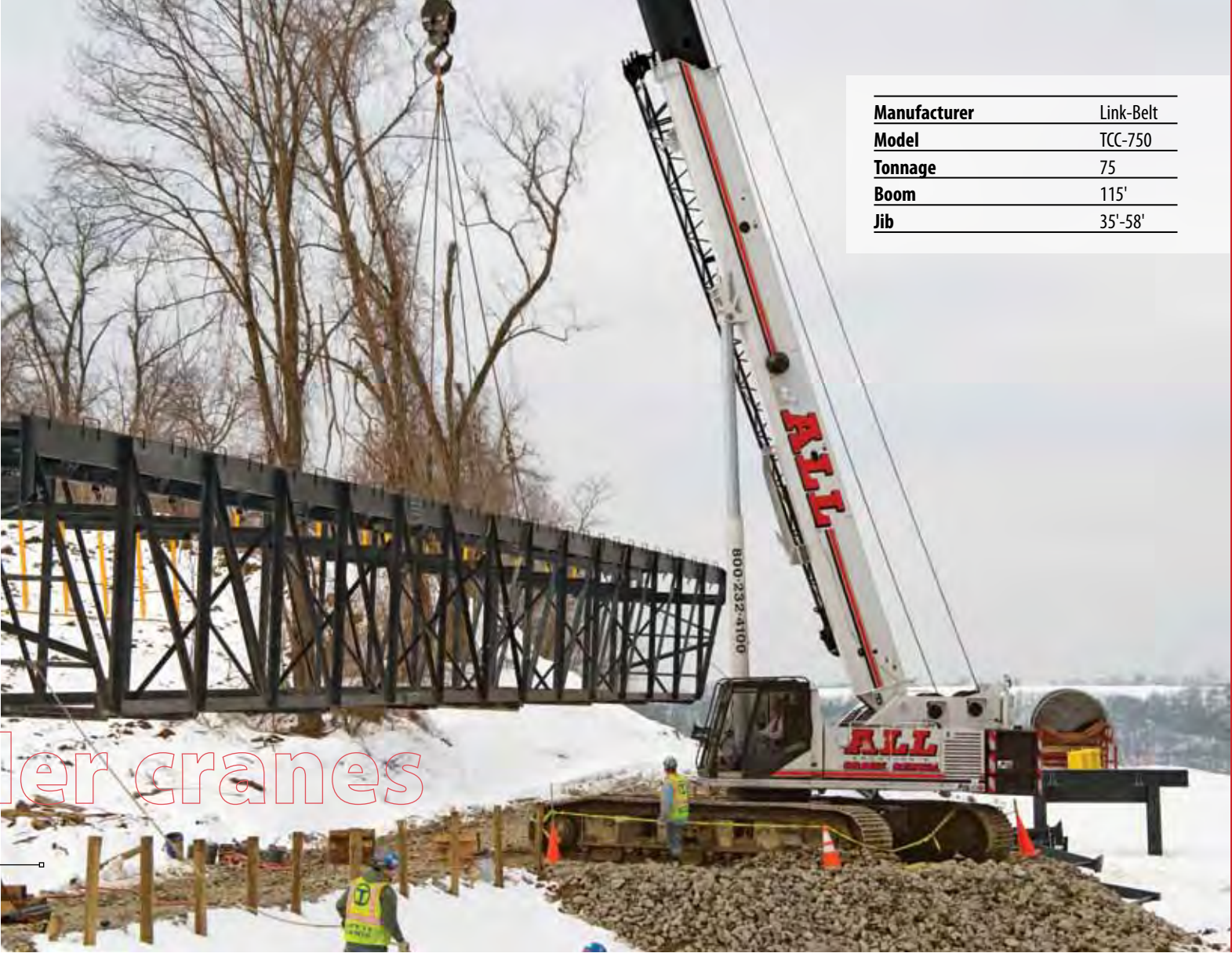
The very first job for the new 75-ton TCC-750: ALL Crane & Equipment Rental Corp. of Nitro, WV, was setting sections of the overland conveyor belt used to transport coal from the mine directly to the prep plant.
