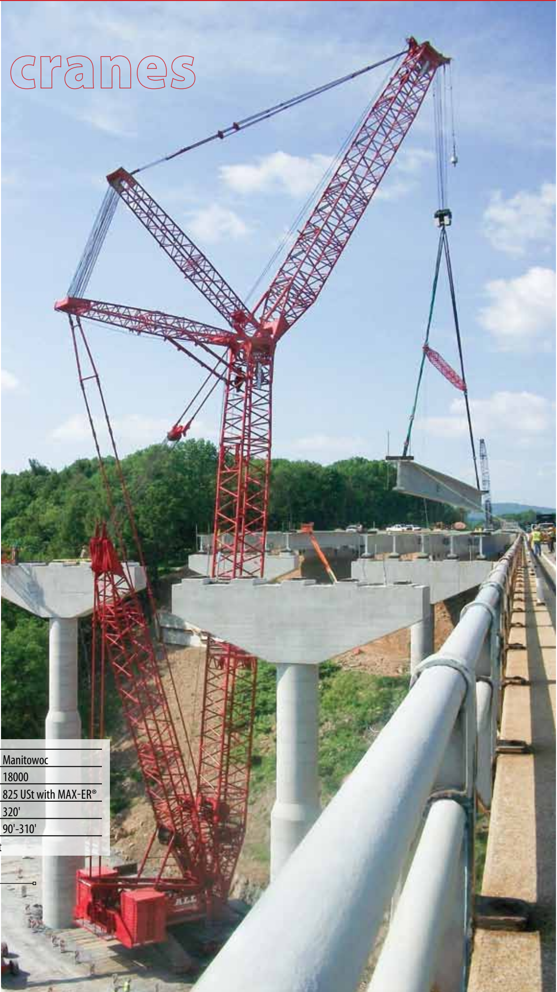
ALL Crane of Pennsylvania used the huge 18000 to set 70 165-ft precast concrete beams more than 100 ft above the Lehigh River and Pohopoco Creek. The crane would have several different configurations during its time on the project, but for its most challenging portion, the 18000 worked with 100 ft of mast, 160 ft of main boom, and a 130-ft luffing jib. It had 528,000 lbs of crane upper counterweight and 320,000 lbs of carbody counterweight.
