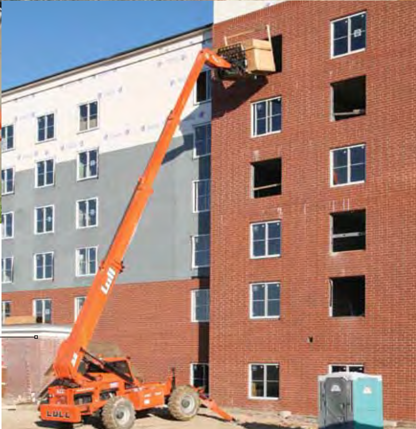
ALL’s new 9,000-lb Lull helping to build the Homewood Suites, Beachwood, Ohio. Fully extended to the sixth floor, this heavy lifter also offers amazing extension, making it a beast on any job site.
