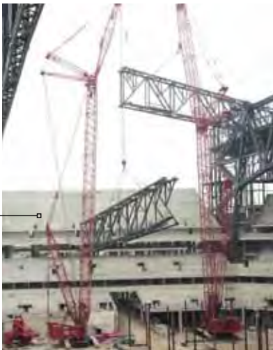
Two Manitowoc 18000s work together setting a roof truss for Lucas Oil Stadium. A wheeled MAX-ER® attachment is sitting to the side but is not attached to the unit. When attached, MAX-ER is a cost-effective way to increase the 18000's base capacity to 825 tons.
