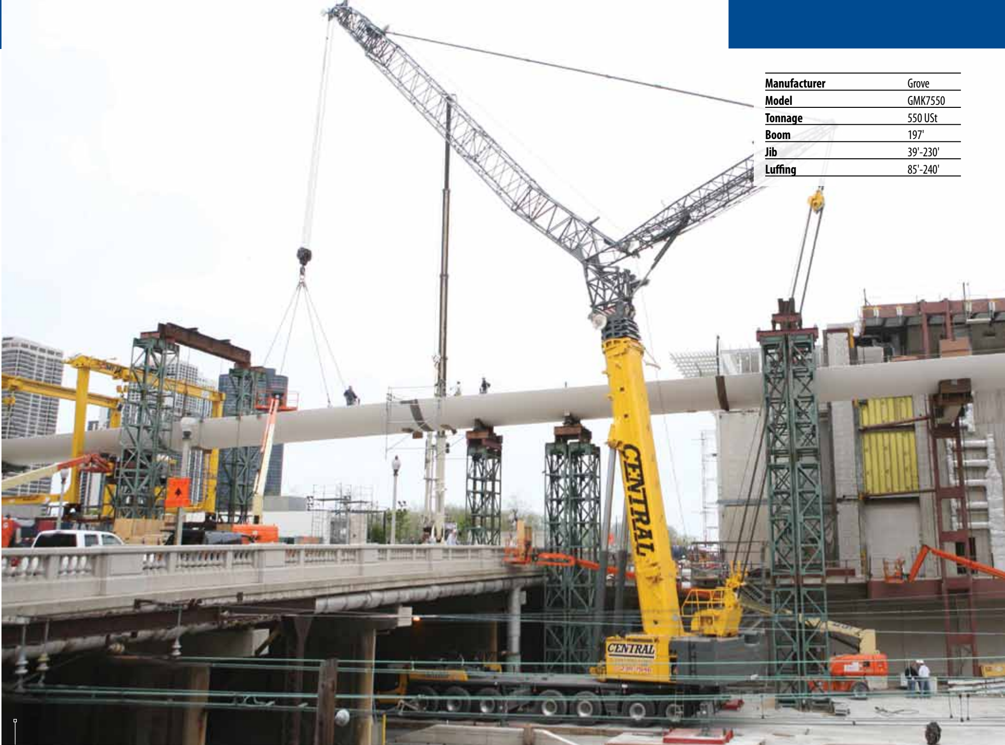
This 7550 helps to erect this steel pedestrian bridge spanning 620 ft from the city park to the third level of a new museum addition. The bridge’s four prefabricated sections—200 tons of structural steel—were hoisted by the GMK7550 and welded together.
