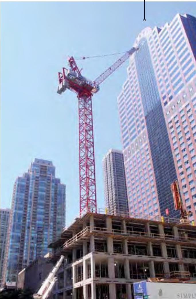
Potain MR 415 luffing tower crane with 164-ft luffing jib; initial mast height 198 ft, final mast height 510 ft. Central Contractors Service of Chicago suggested the use of the MR 415 for its extremely high line speed.
